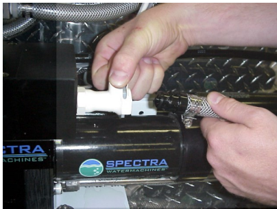
Connecting brine discharge service hose
